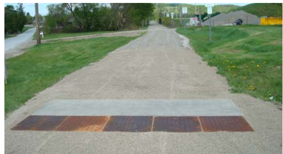
Newly installed truncated dome
